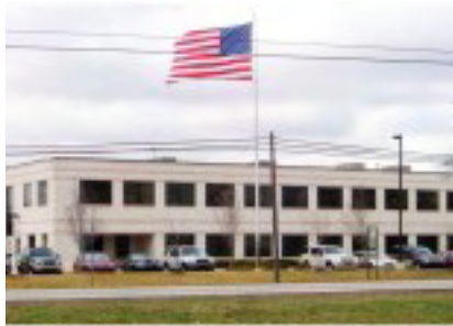
Western Waterproofing: Livonia, MI
